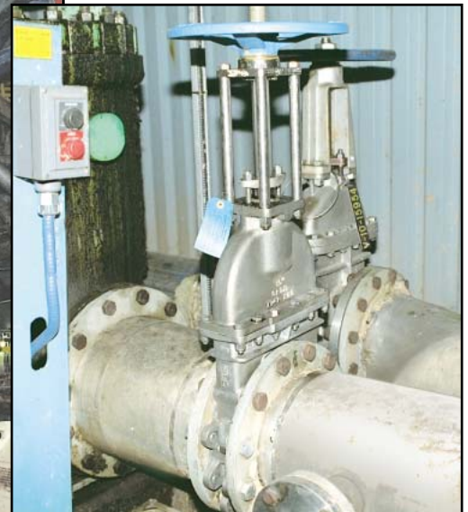
Filter isolation installation.
